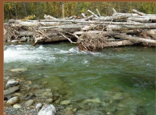
An engineered log jam at the restoration site on Moose Creek.
