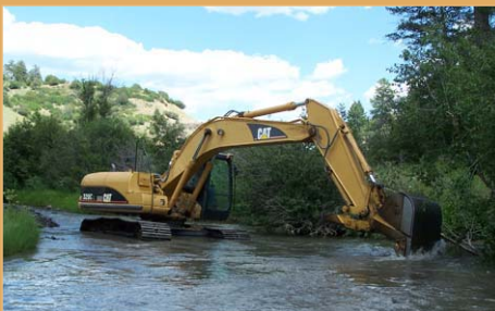
Tools of the trade. Eudane Vicenti of the Jicarilla Game and Fish Department uses an excavator to establish and enhance complex pool habitat for the benefit of the Roundtail Chub during a 2009 Habitat Project on the Navajo River, Dulce, NM.
