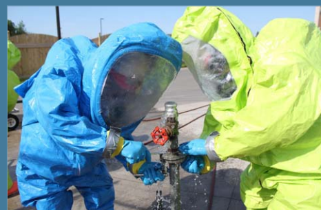
Repair of damaged equipment
